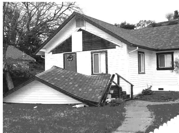
Figure 6 - San Simeon Earthquake, Dec. 22, 2003 The collapsed porch was not adequately attached to this single family residence.
