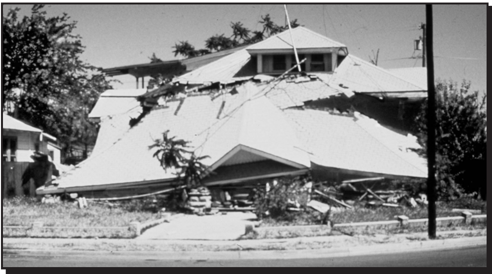
Additional damage from aftershocks
